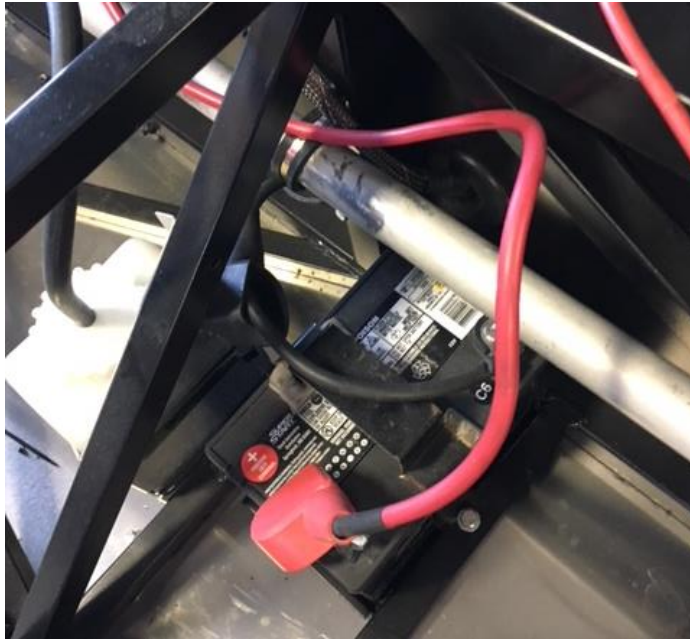
Figure 36 – Battery Cable Installation
