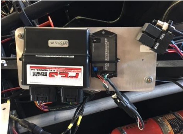
Figure 34 – ECU, Relay, and Wide Band Mounting (Underside View)
